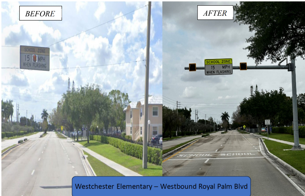
Figure 4: Example of Single-to-Dual Overhead Flashing Beacon Conversion
